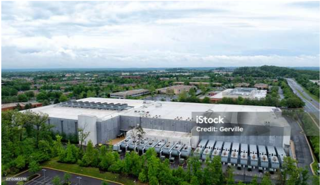
Figure 1. Aerial view of a data centre in Sterling, Virginia.
