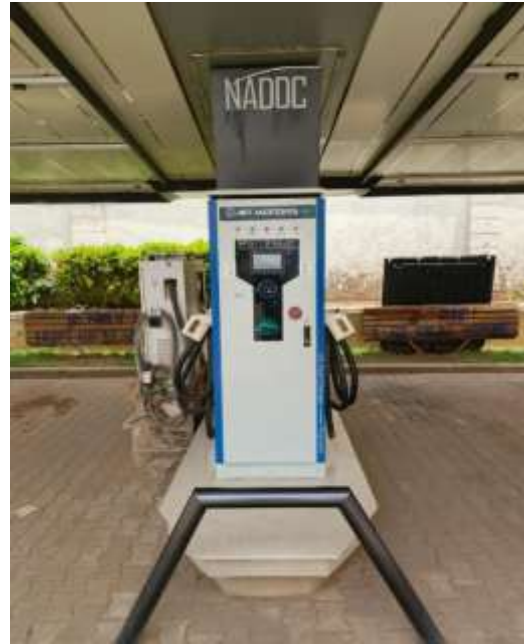
Plate A4: Level 3 Charging System
