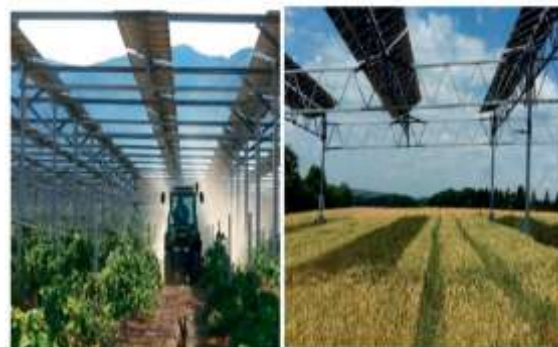
Figure 3 (b): Photographs of operational agrivoltaic systems in the field. The images show elevated solar panel arrays with crops growing underneath and sufficient clearance for tractors and other agricultural machinery to move freely [13].
