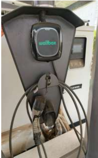
Plate A3: Level 2 Charging System
